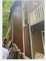
weatherboards on a house with very similar-looking fibre cement boards: because of woodpeckers. Both sides of the house with timber had been attacked by those destructive birds, leaving dozens of holes in the timber (Aussies living near flocks of cockatoos can empathise!) – fibre cement boards, however, are impervious to woodpeckers.
